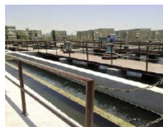
Concrete repair of the clarifier at Naga Hamady WTP, Qena, Upper Egypt
