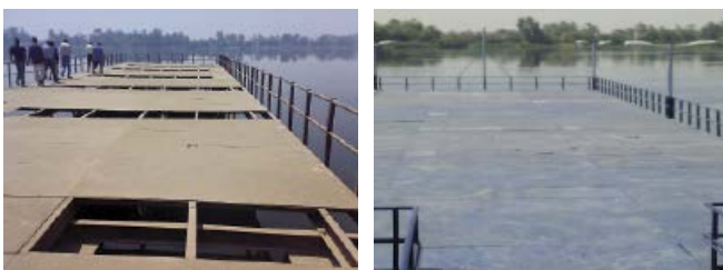
River Intake flooring replaced, Dishna WTP, Qena, Upper Egypt
