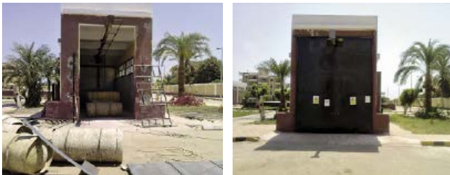
Securing the Chlorine Drum Store, Dishna WTP, Qena, Upper Egypt
