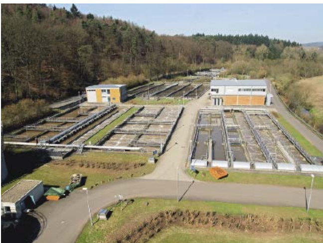
Fig. 1: Aeration basins in Kaiserslautern
