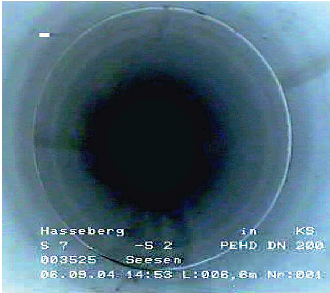
Fig. 5: Reality: Camera inspection of the sewer: hydraulically smooth pipe joint
