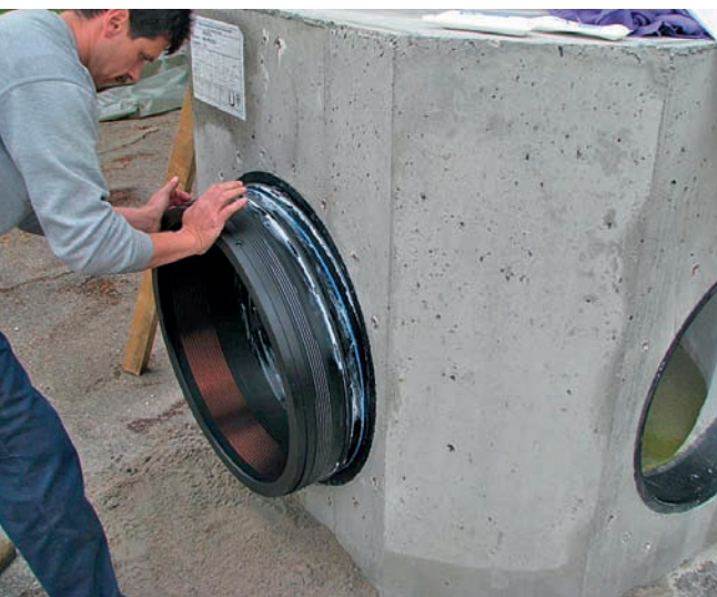
Fig. 11: Connection of PE pipes to a concrete man whole base with sewage inspection chamber lining ASF and insert sleeve AEM
