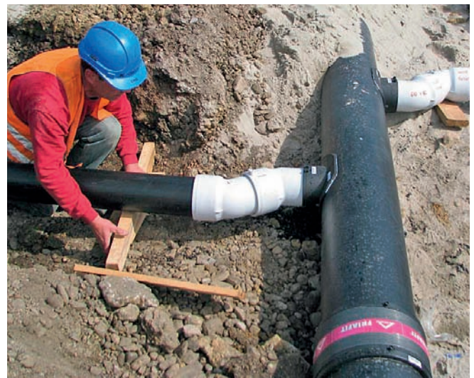
Fig. 13: Domestic sewer pipes are connected using the sewage saddle ASA-TL, in this case in connection with sewage elbows ABMS d160
