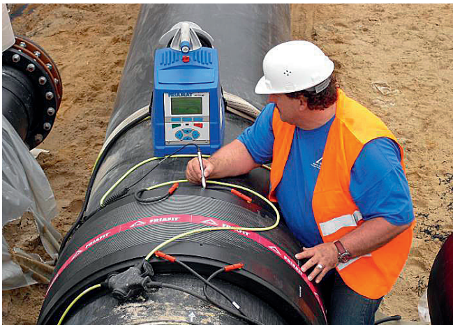
Fig. 6: PE pipe, joining method: electrofusion welding, coupler and electrofusion unit
