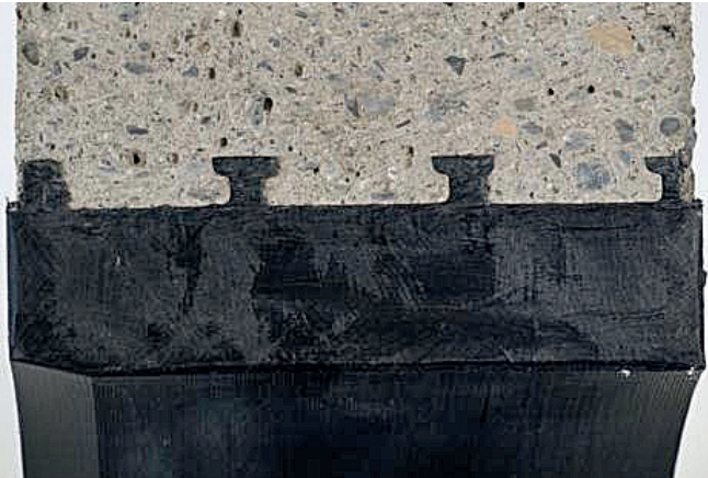
Fig. 10: The undercut anchoring webs of the inspection chamber lining ASF provide a strong and tight connection to the concrete.
