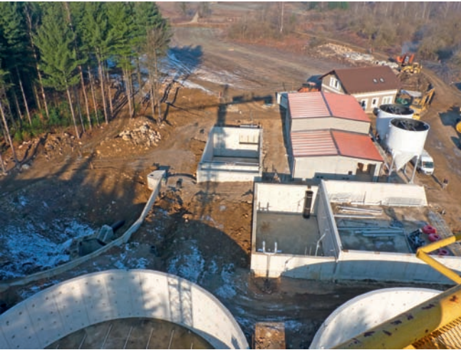
Fig. 2: Water and wastewater treatment plant Ogulin under construction
